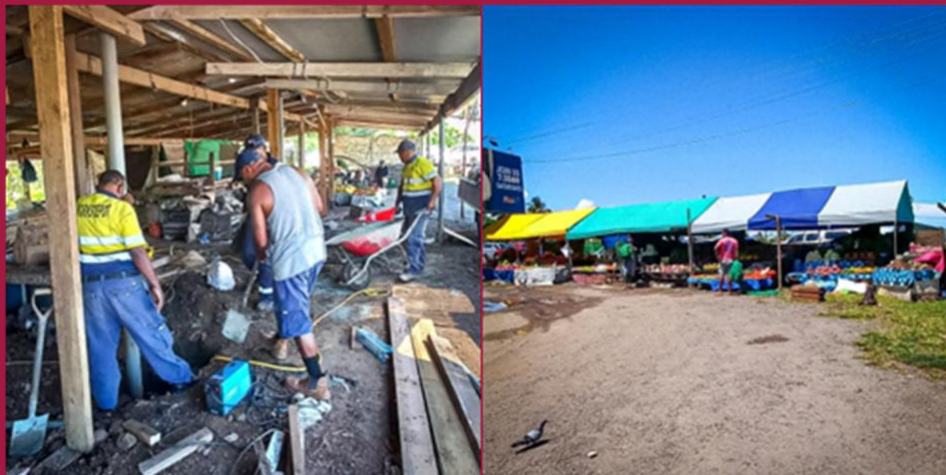
Figure 19: Renovation work of the Raiwaqa Market
