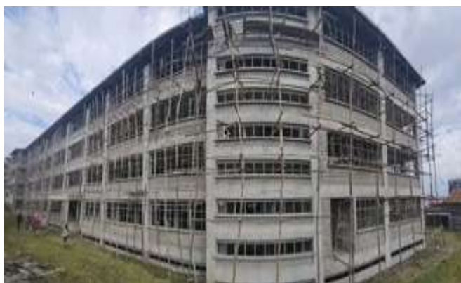
Figure 32: Bondeni Affordable Housing Units
