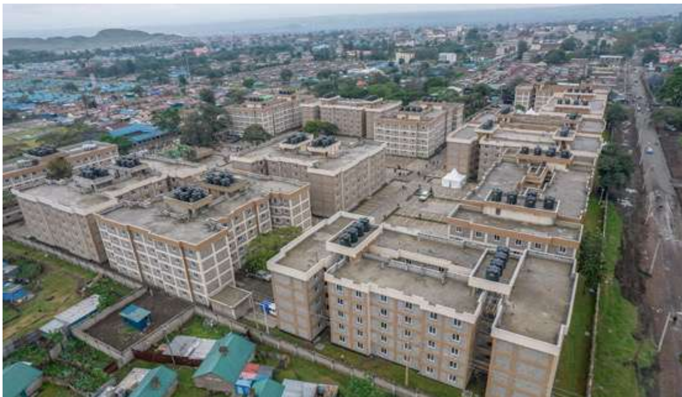
Figure 29: Bondeni Affordable Housing delivered 605 units and launched in January 2024
