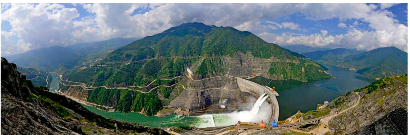
Figure 5.25 View of Xiaowan Hydropower Plant
