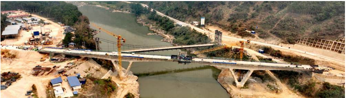
Figure 5.52 On April 12, 2023, the China-aided Kunlong Bridge in Myanmar was successfully connected
