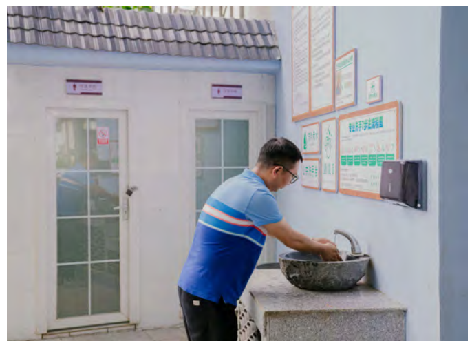
Figure 5.23 On-street public toilets in Qinghua Community, Linxiang District, equipped with handwashing facilities and promotion materials
