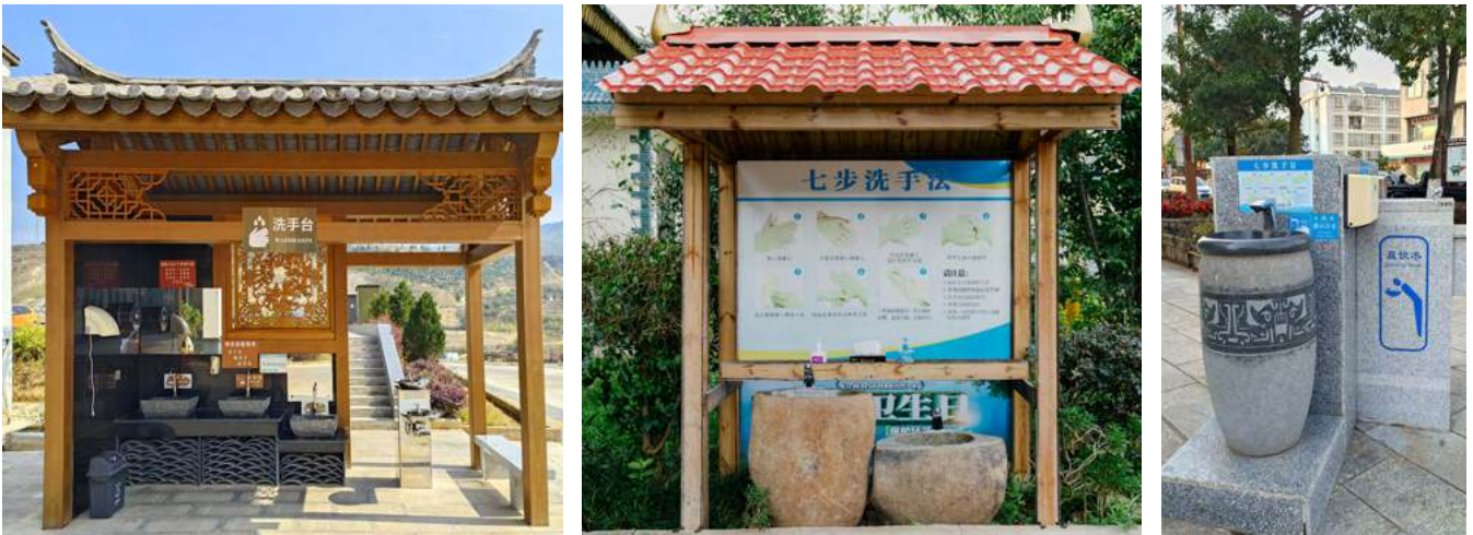
Figure 5.22 Handwashing facilities in public places with promotion signs
