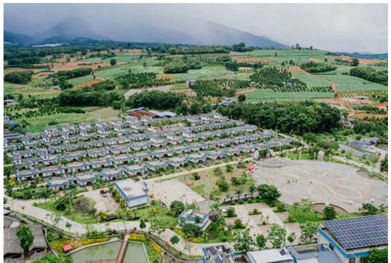
Figure 5.4 Aerial view of Ze’an New Village, Hepai Township, Gengma Autonomous County
