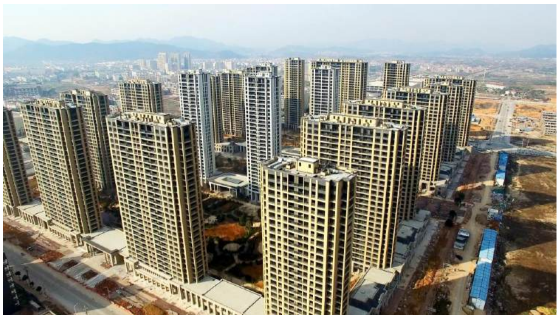
Yiwu New Community Construction
