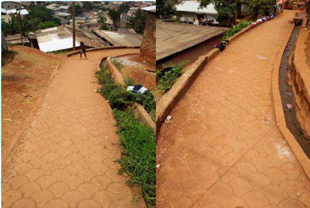
Figure 7: View of a slum track developed in the Ngoa-Ekélé district in Yaoundé
