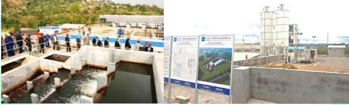
Figure 2: Water treatment plant through PAEPYS
