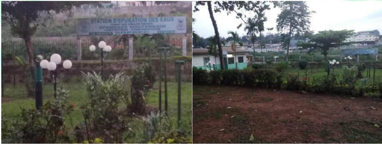
Figure 5: wastewater treatment station of the camp sic MESSA in Yaoundé
