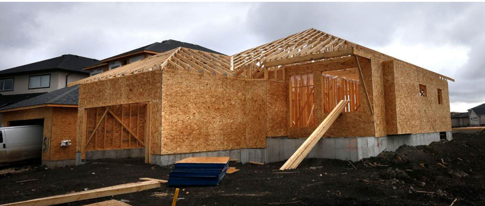
New house construction in Winnipeg. (Wayne Glowacki / Winnipeg Free Press / September 12, 2016.)
