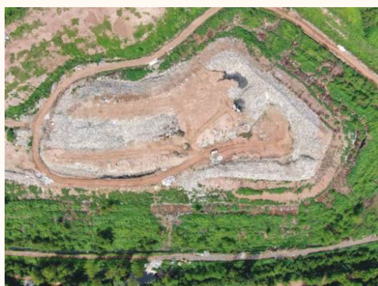
Figure 30 Udon Thani City Municipality Landfill
