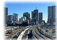
Loop road 2 (between Tsukiji and Shimbashi)
