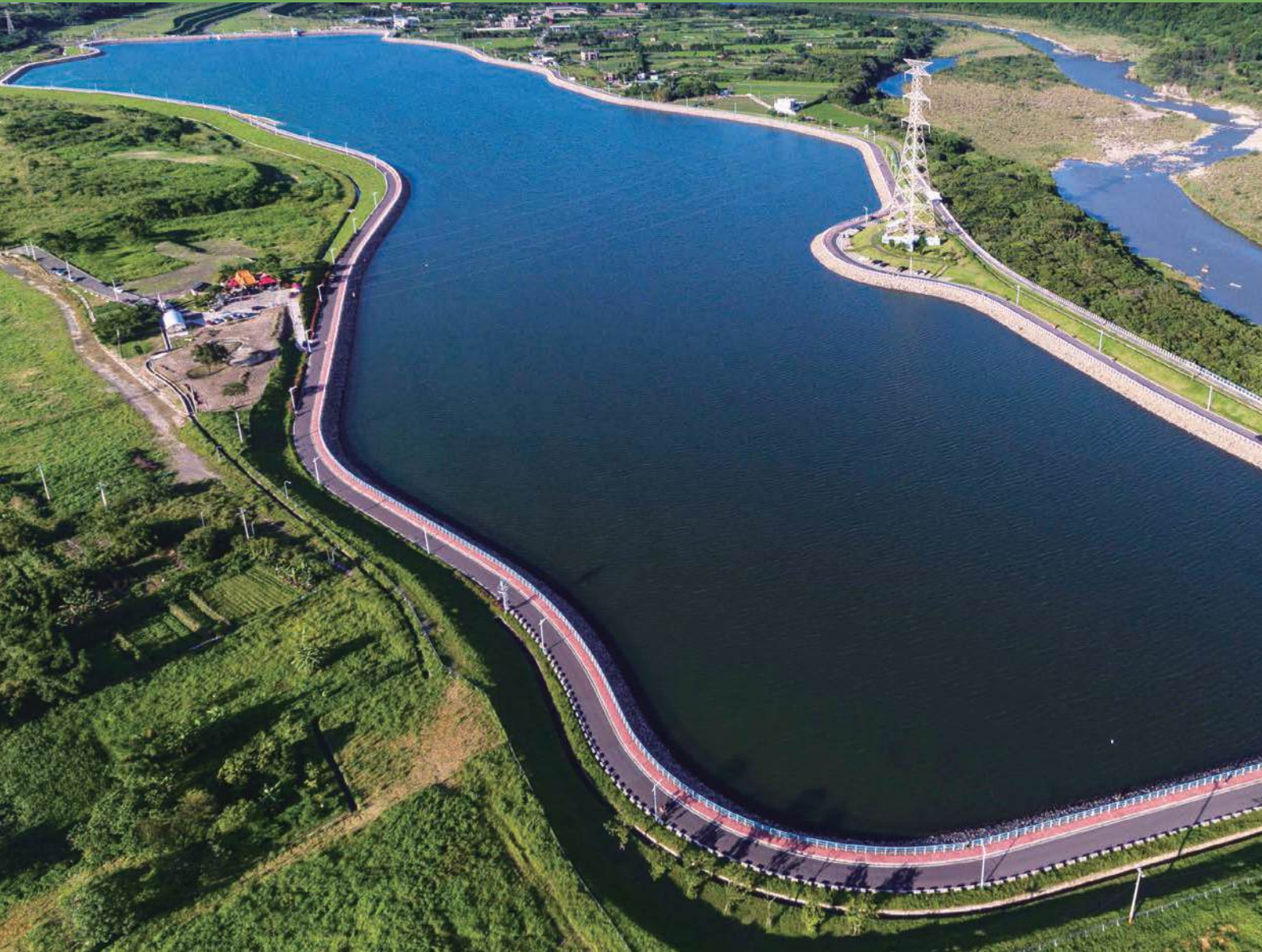
Daxi Zhongzhuang Adjustment Pool and Peripheral Trails / Credit: Northern Region Water Resources Office, Water Resources Agency, Ministry of Economic Affairs
