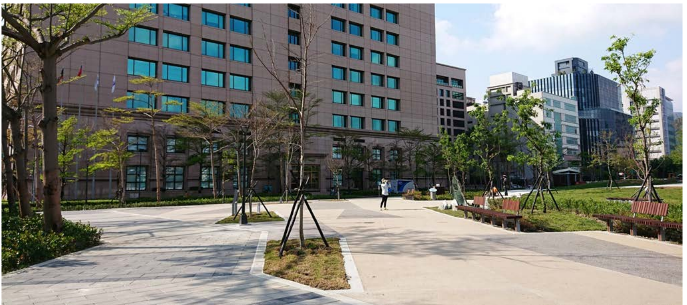
► Water-permeable sidewalk at Gangqian Park.
