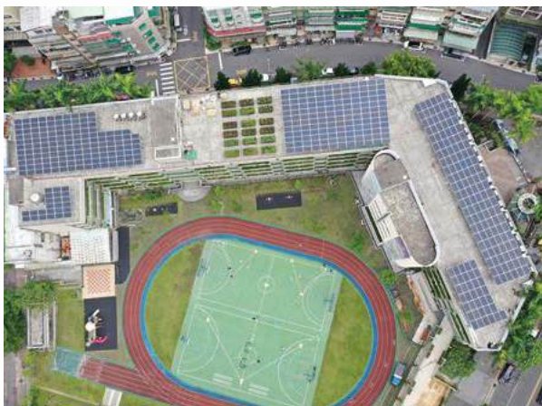
▶ Installation of 146.4kW at Wan Xin.
