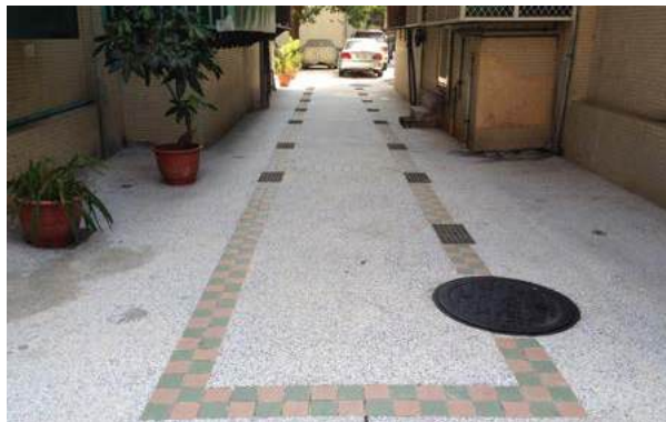
► Post-construction of user drainage equipment project for sewage.
