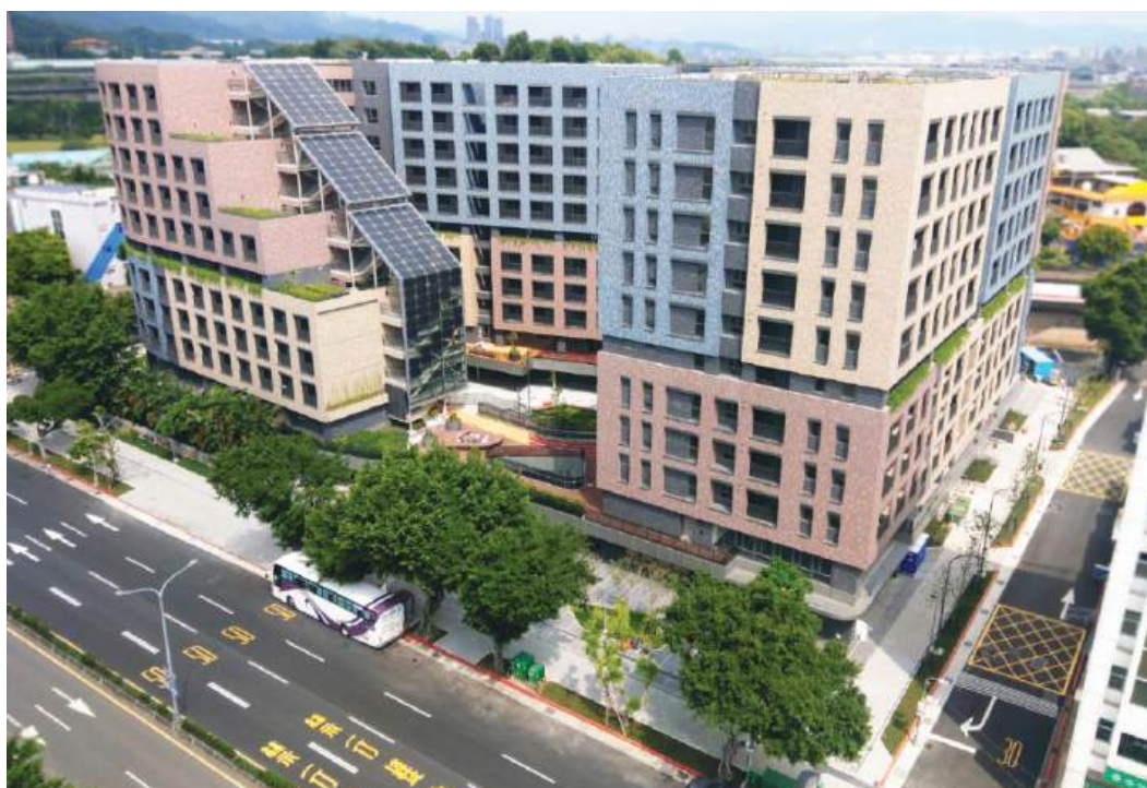
▲ Construct diversified social housing - Minglun Social Housing
