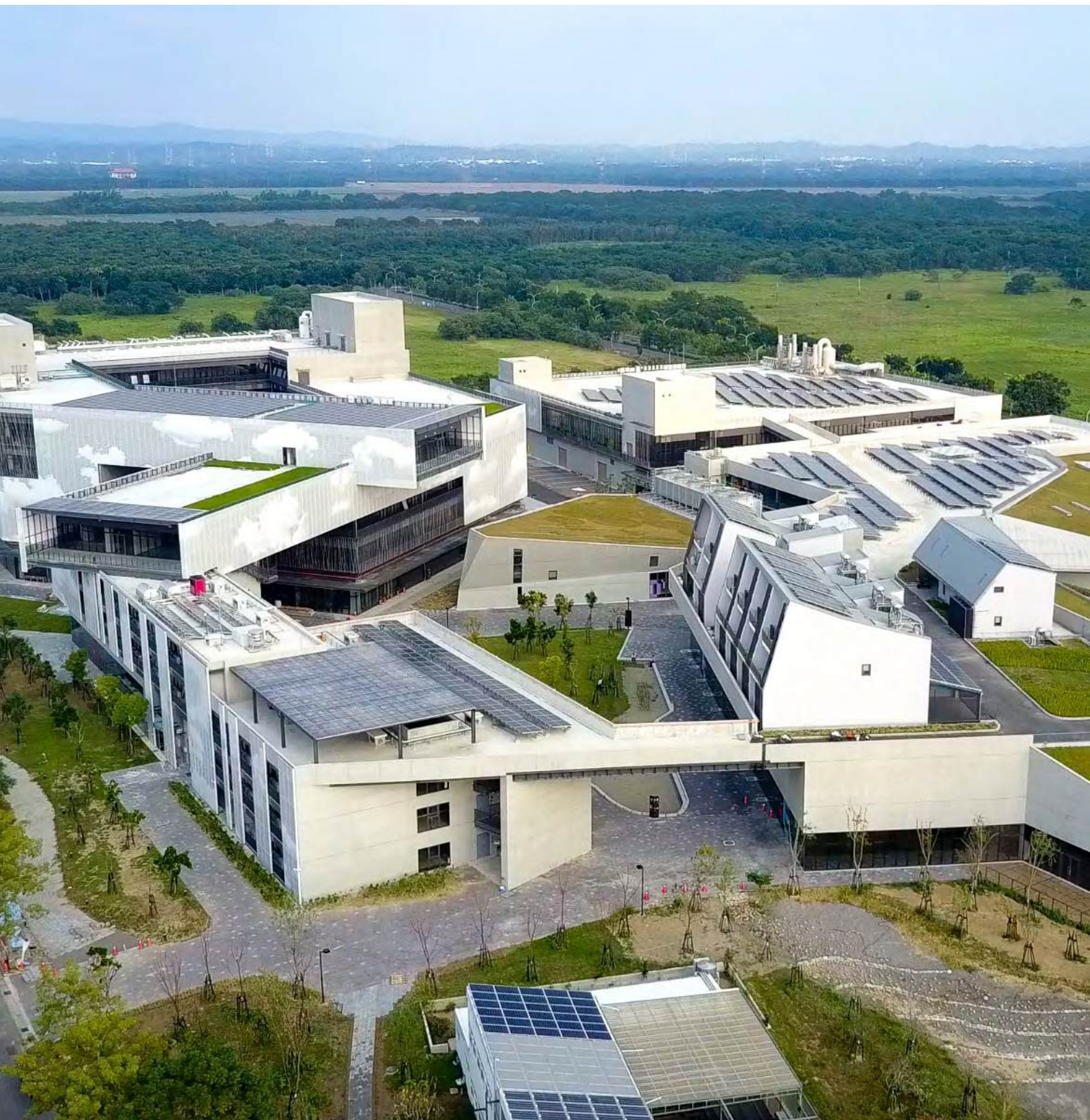
△ Shalun Smart Green Energy Science City
