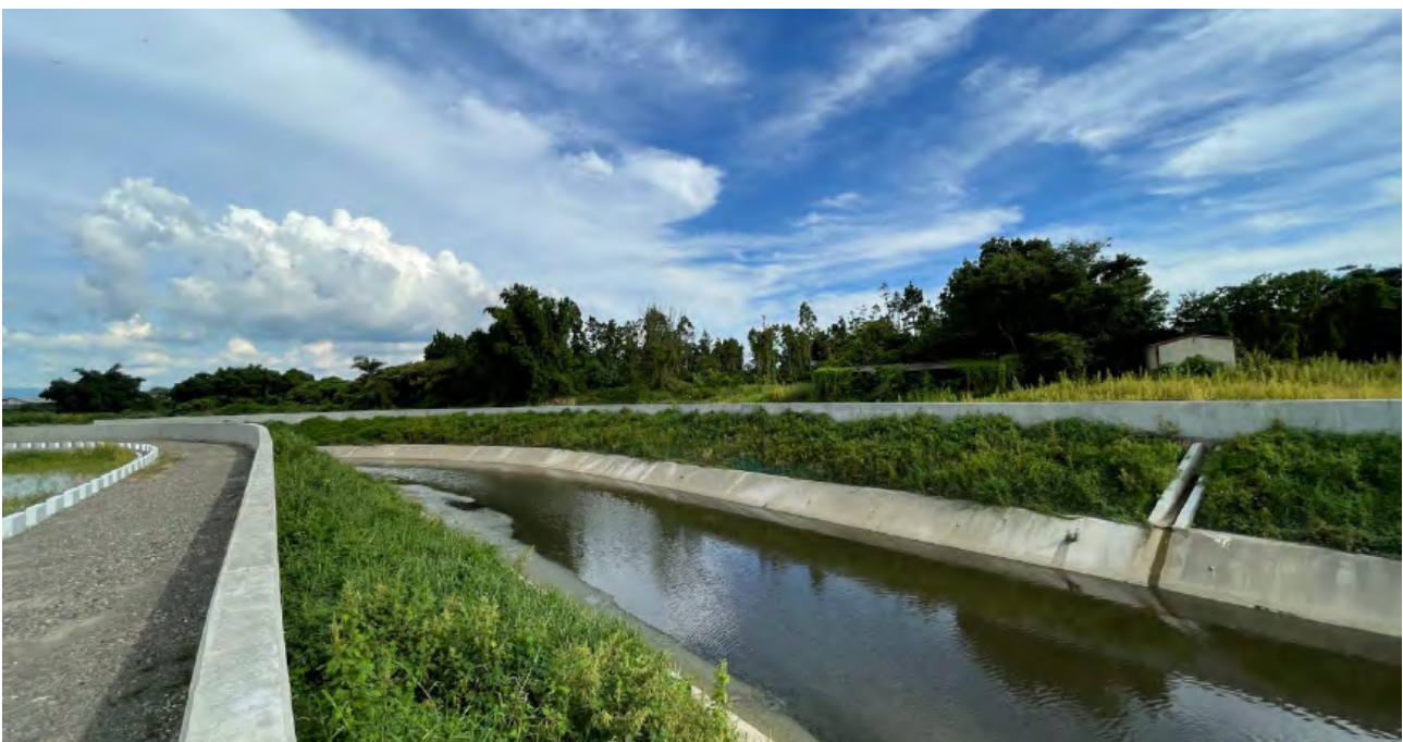
△Gueizi Harbor Drainage Shoreline Treatment Project (3K+943~4K+241)
