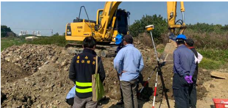
△ Supervision of Site Pollution Remediation
