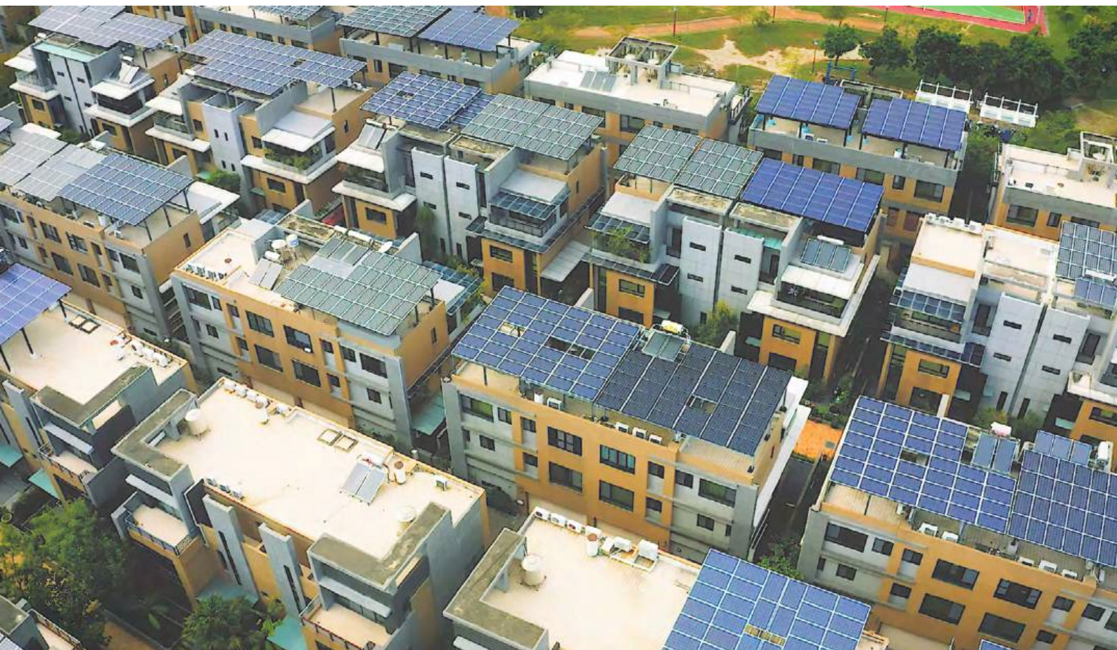
△ Green Roofing in Tainan City's Annan District
