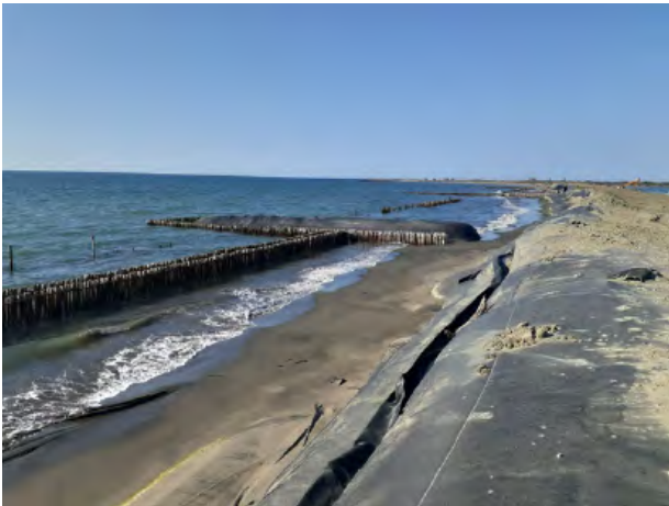
△ Bamboo Piles and Sandbags Replace Concrete to Reduce Carbon Emissions
