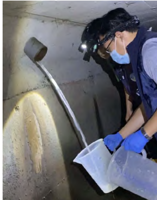
△ EPB Sewage Inspection
