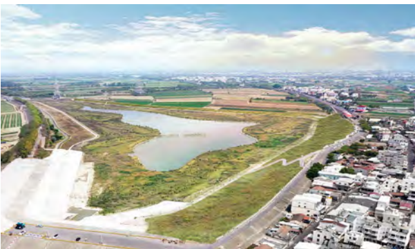
▲ Sucuo Flood Detention Pond - the largest flood detention pond in Tainan
