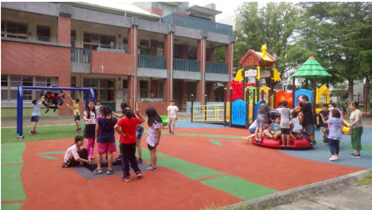
▲ Installation of inclusive playgrounds in schools
