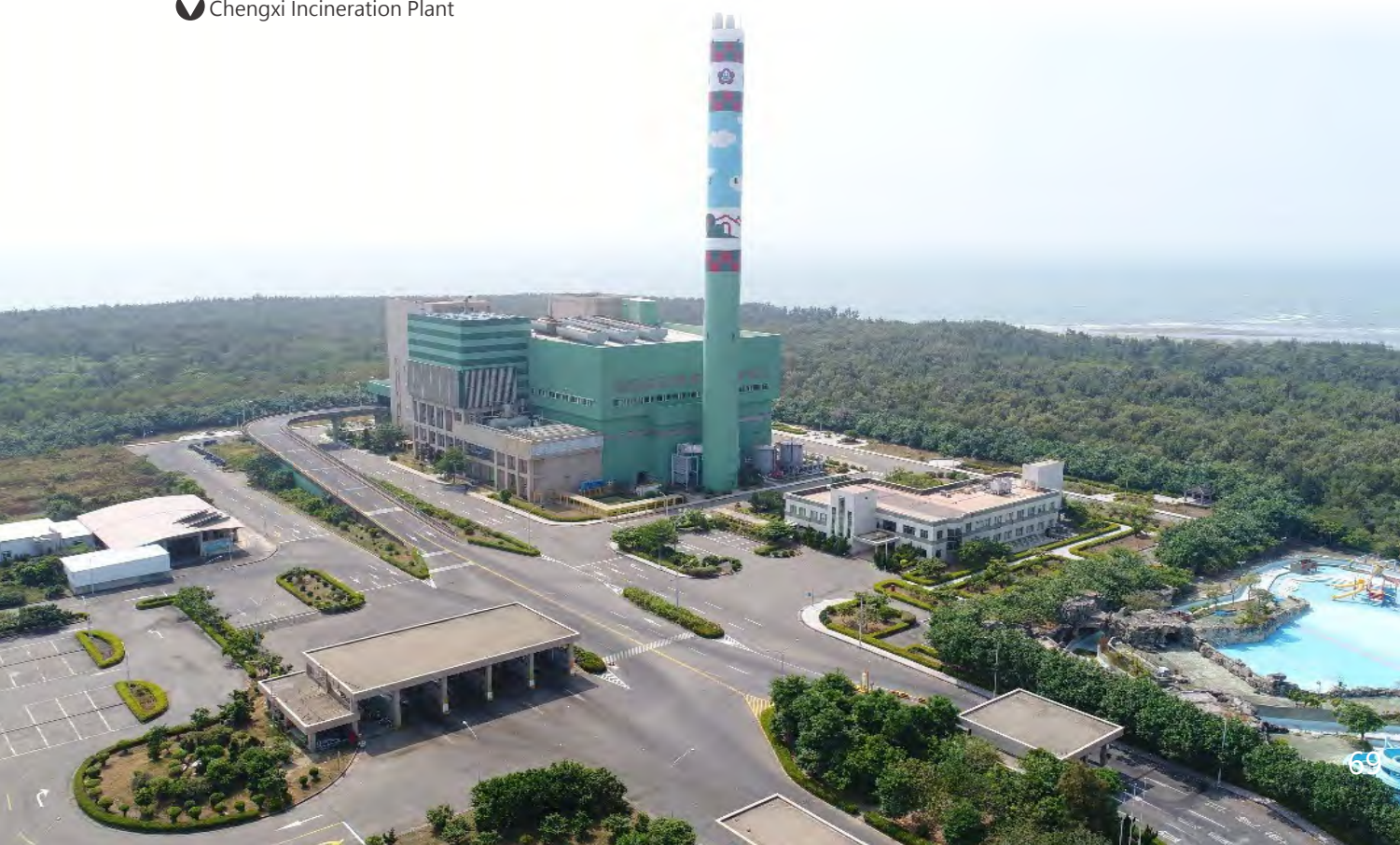
▼ Chengxi Incineration Plant
