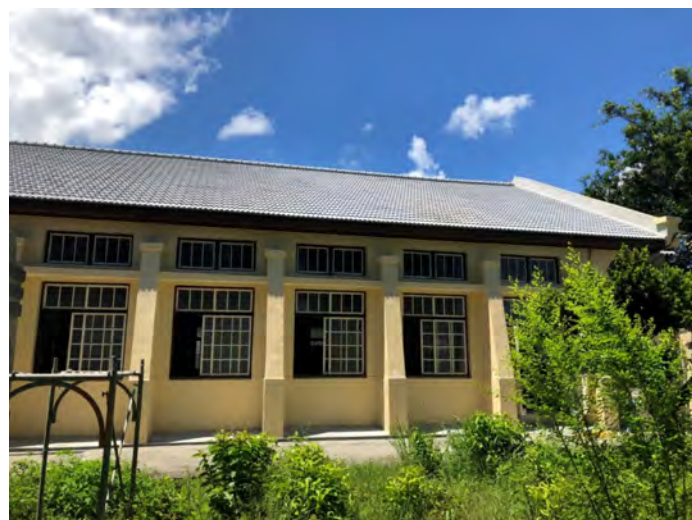
▲ Restoration for the Original Auditorium and Clock Tower Base of the Yanshui Huanya Elementary School: Restoration work for 88 Sash Glass Windows in the Auditorium
