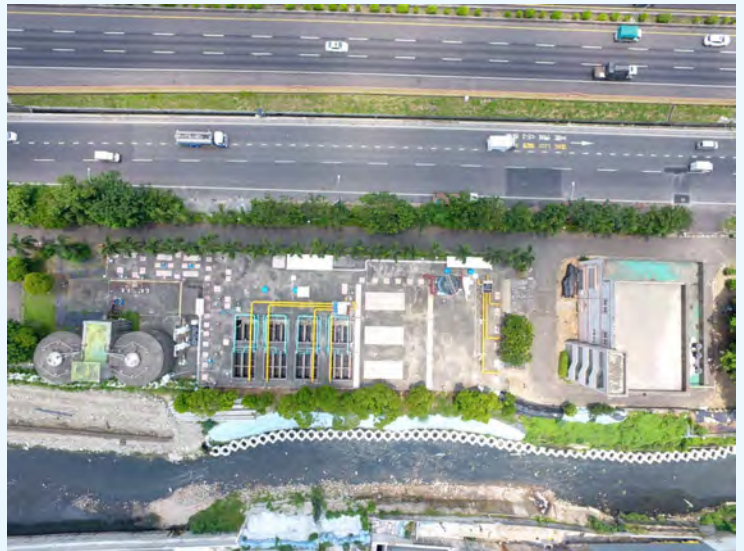
▲ Aerial photo of Sanye River
