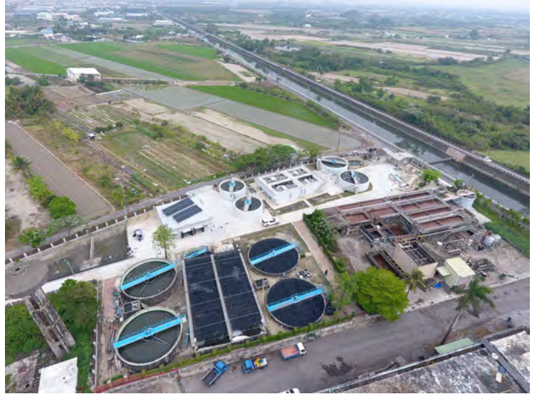
▼ Anshun Drainage Water Purification Plant
