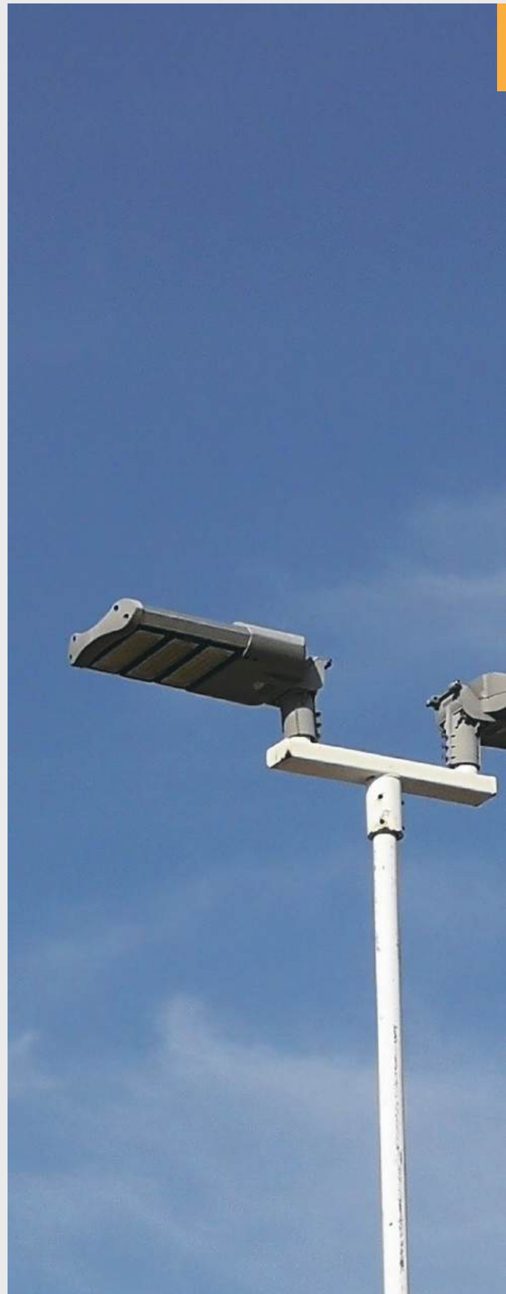
▲ Undergoing the replacement of the LED light
