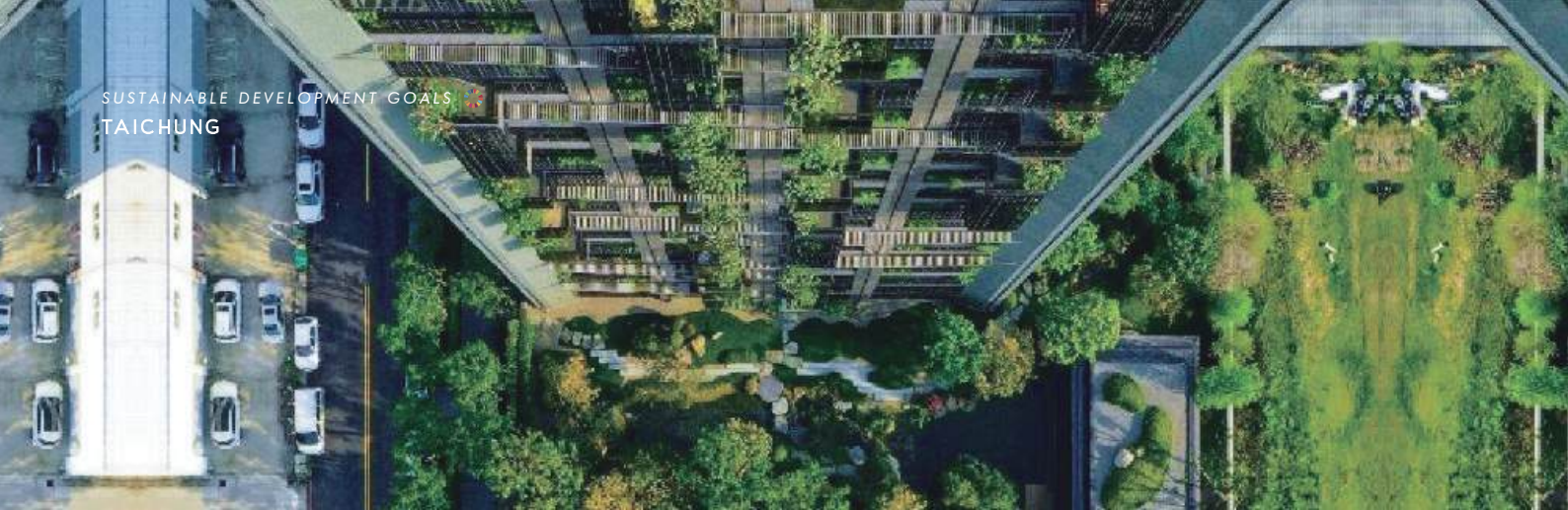
▲ Vertical greening of building façade
