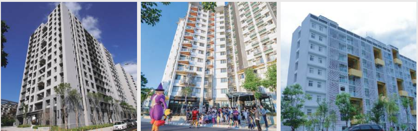
▲ Nantun District Jingke Lohas Good House, Fengyuan Ankang Phase 1 Council House, Dali Guangzheng Section Community House Phase 1.
