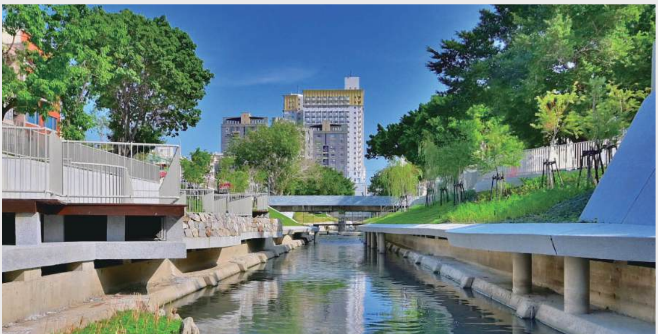
▲ After rectification of Liuchuan Canal, it is the first landscape river bank in Taiwan with a low-impact development design.
