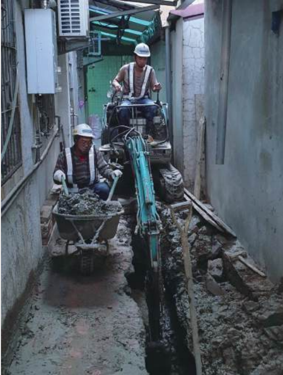
▲ The ongoing construction for sewage project in West District
