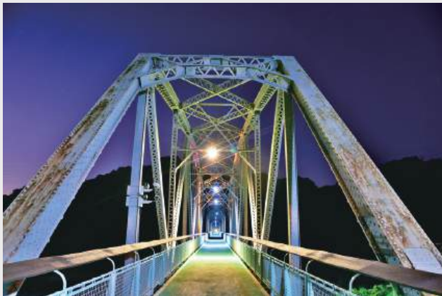
▲ Houfeng railway steel beam bridge
