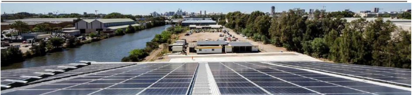
Alexandria Canal Depot: PV Solar Installation
