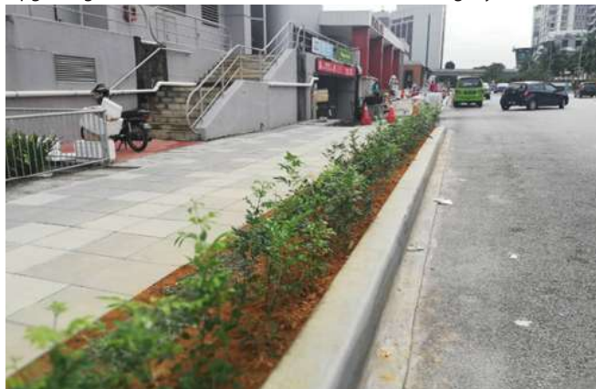
Upgrading work for barrier-free infrastructure in Subang Jaya
