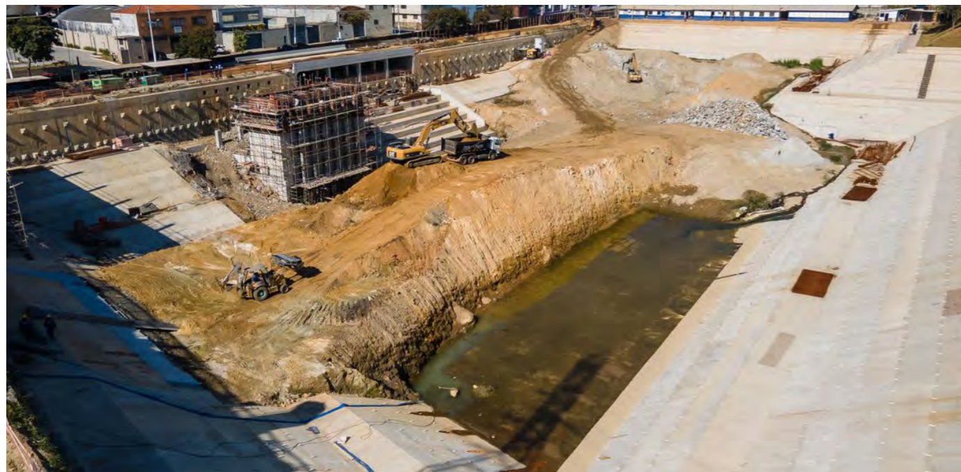
Construction of the Taboão swimming pool on Aricanduva Avenue.
