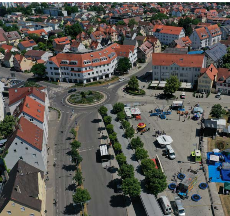
Photo 24: Green moat and bus station, Source: City of Rottenburg
