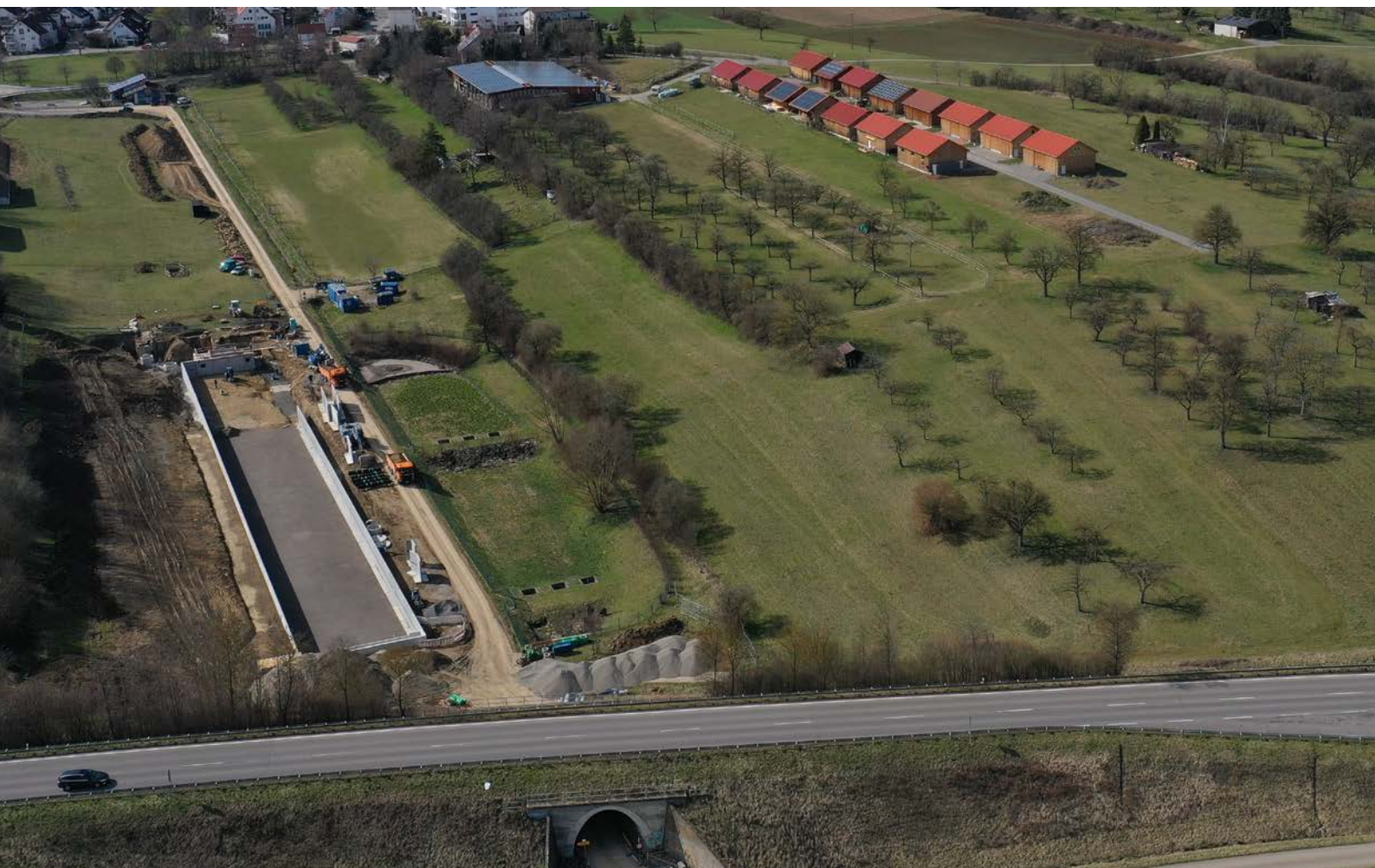
Photo 14: New construction of retention soil filter AZV Bondorf/Hailfingen
