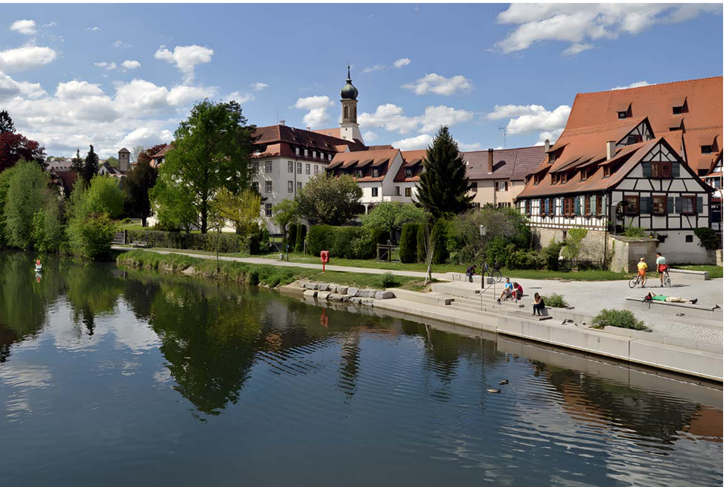
Photo 6: Rottenburg House Nepumuk on the Neckar River, Source: Rottenburg City Council
