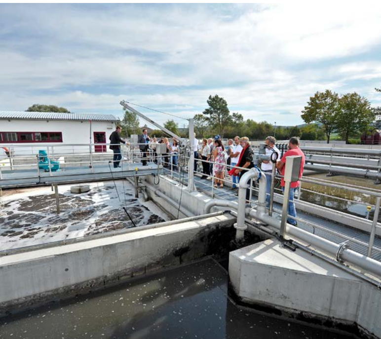
Photo 12: Trial start-up-EssDe_Wastewater_treatment_plant-Kiebingen, Source: Municipality of Rottenburg
