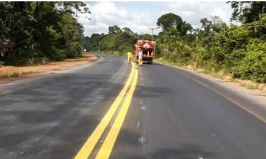
ROAD CONSTRUCTION Requalified stretch of PA-483, and requalification of PA-483.
