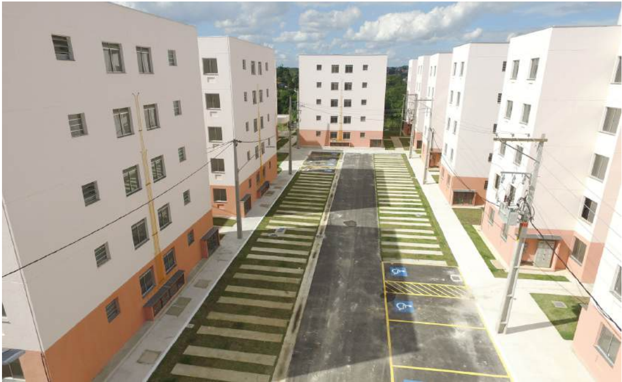
New housing units built.
