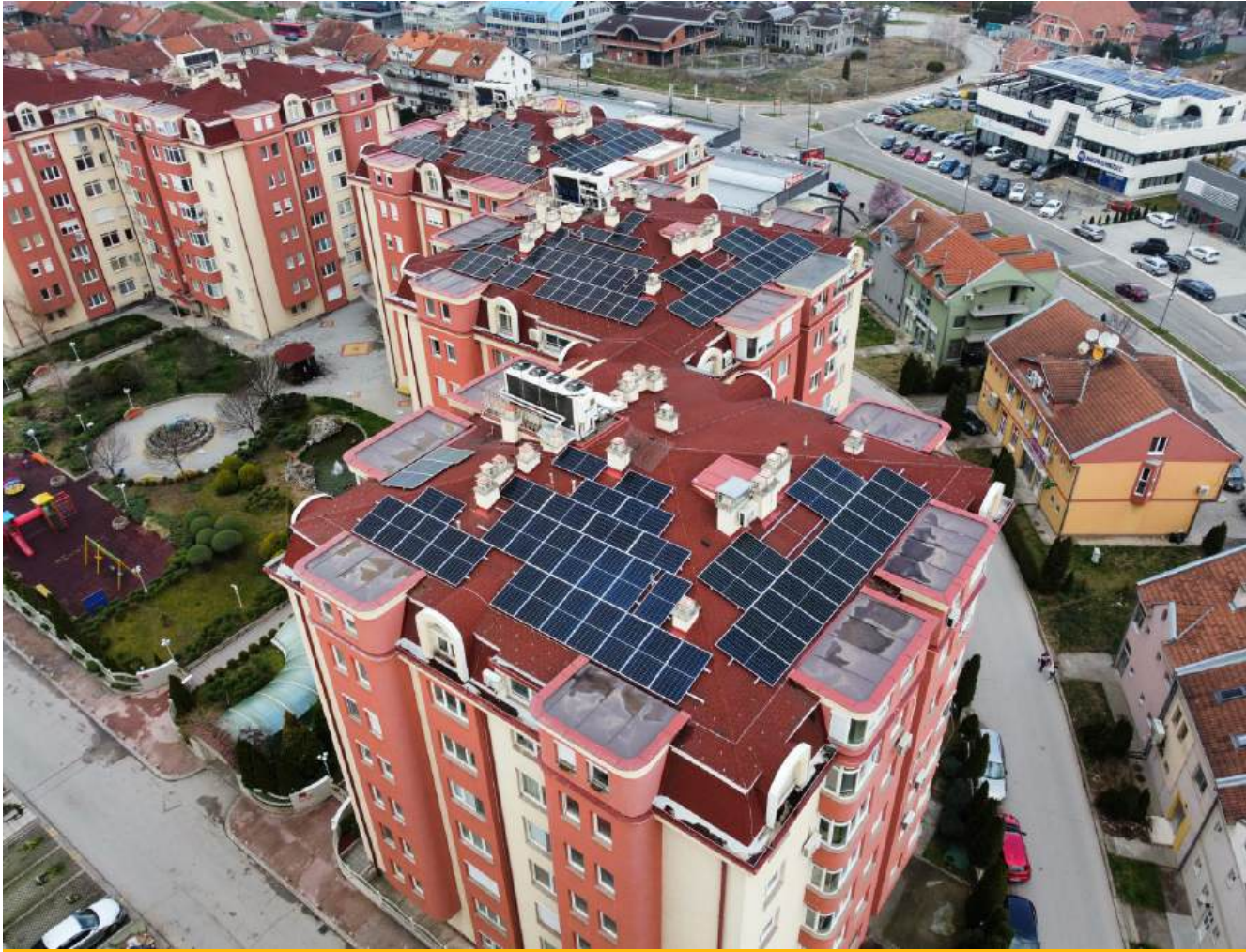
Figure 26. Residential complex Magdon Niš with solar panels installed on the roof. Source: Energy Manager of the City of Niš, Center for Sustainable Energy Development – CORE Niš.
