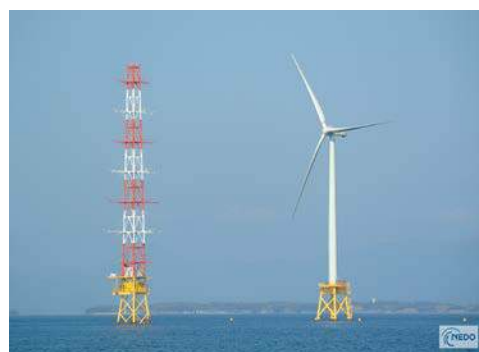
Wind power generation
