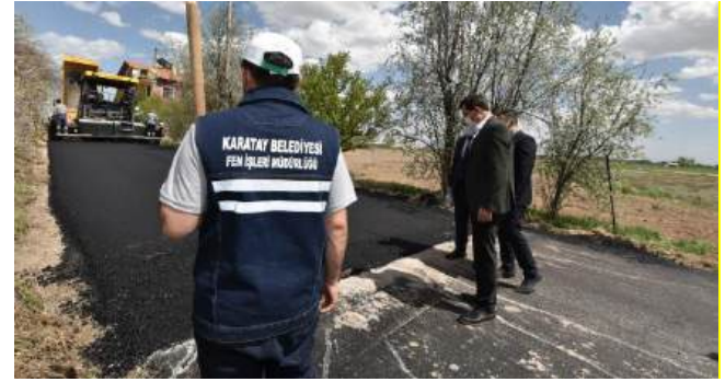
Image 11: Asphalt construction in the city center of Karatay
