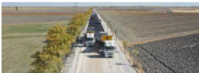
Image 10: Asphalt constructions in the suburbs of Karatay
