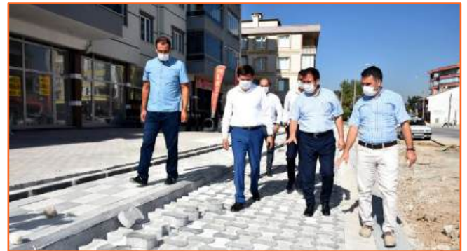
Image 54: Kerbs installation works in Karatay
