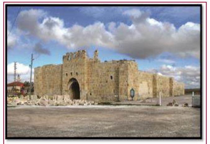
Image 51: Restoration of Obruk Inn
