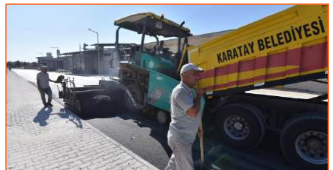
Image 55: Paving works in Karatay
