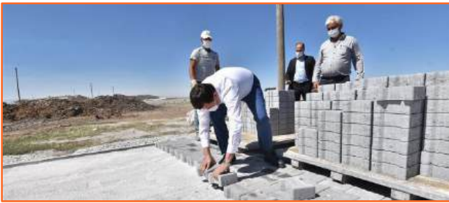
Image 52: Street paving works
