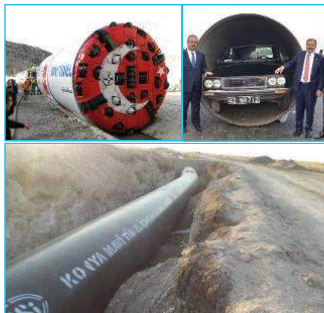
Image 39: The “Blue Tunnel Project”
