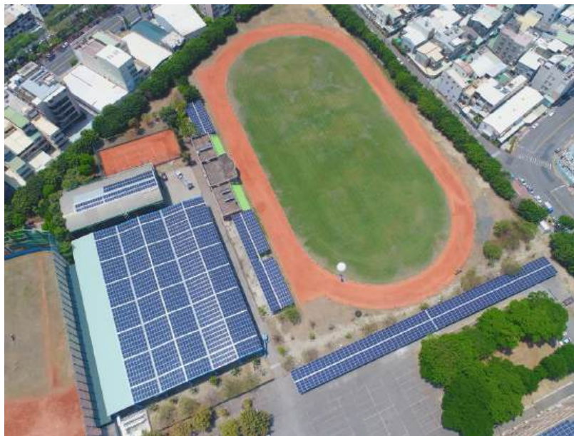
▲ Photovoltaic projects on campuses
