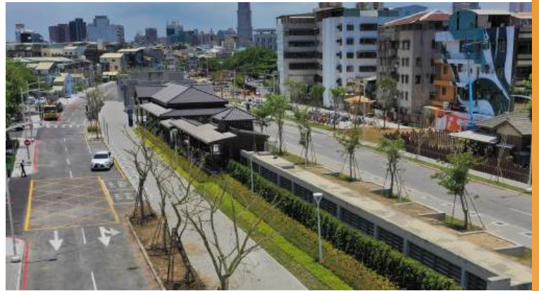
▲ Underground Railway Project
