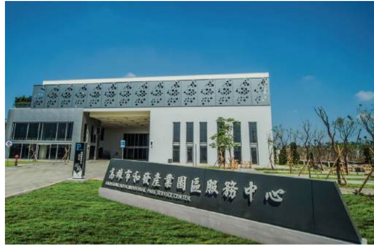
▲ Hofa Industrial Park Service Center
