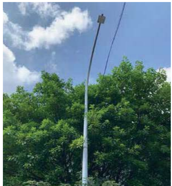
Replace 3 sets of LED85W fixtures in Lane 118, Sec. 1, Yanping Road
