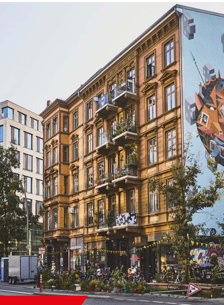
Photo 45: View of the Gängeviertel © Mediaserver Hamburg / ThisIsJulia Photography
