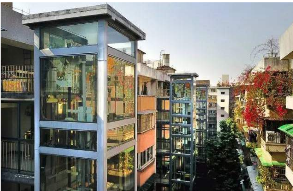
Installation of elevators in existing buildings
