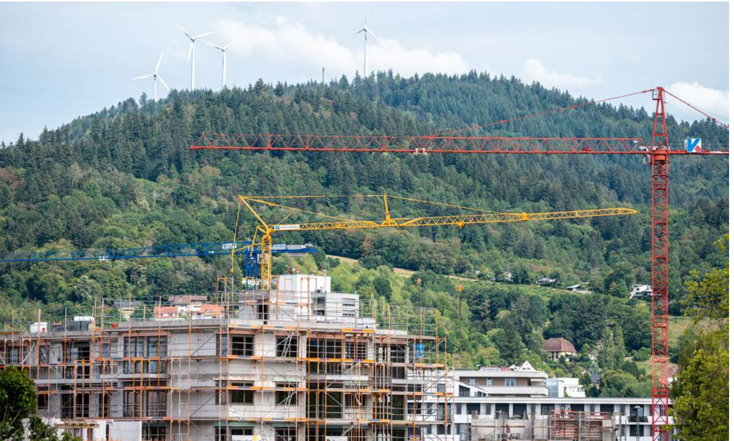
Photo 22: A construction site in Freiburg © Stadt Freiburg
