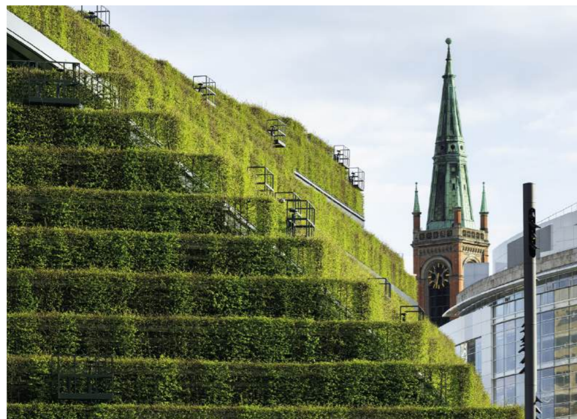
PHOTO: Green facades and roofs in the densely built-up inner city - climate adaptation to protect against heat
