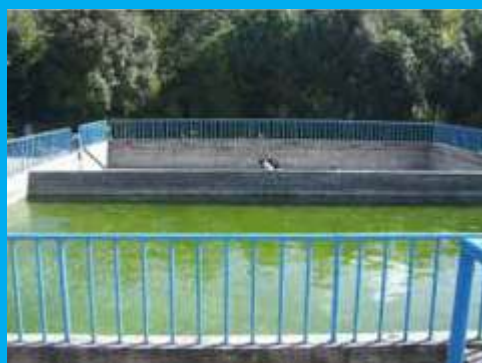
Figure 21: Drinking water treatment plant
