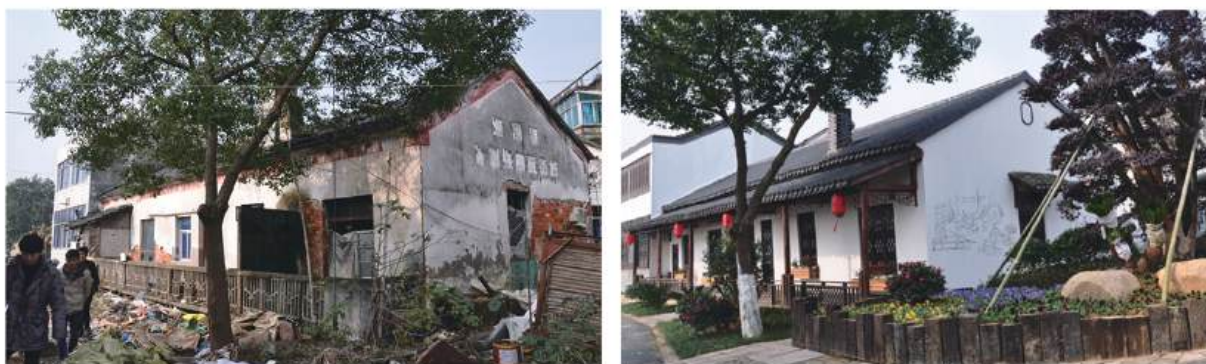
Fig. 2-27 Comparison of the Dangerous Housing Before (left) and After Renovation (right)
