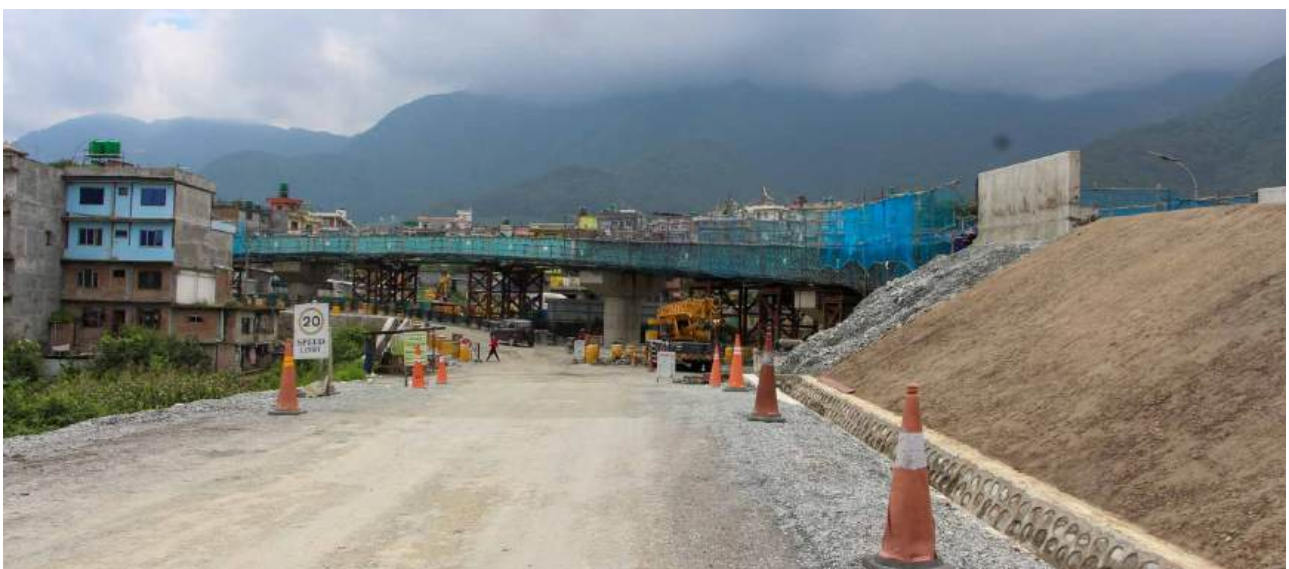
Flyover under construction phase © UN-Habitat, 2024
