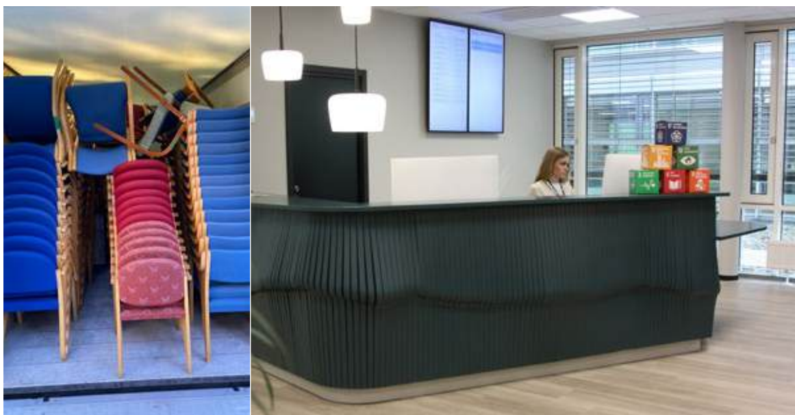
Reception desk made by discarded chairs. The seats and backs of the chairs are turned into sound attenuation elements.
