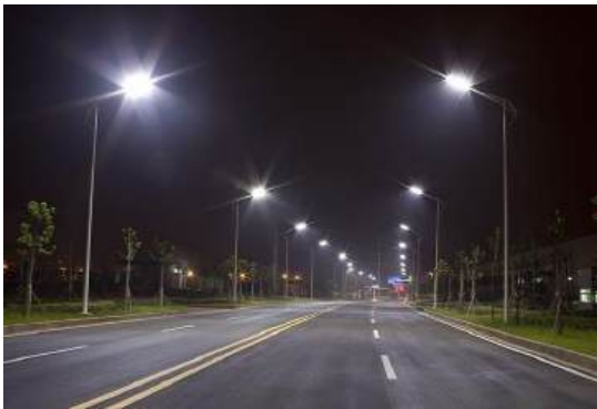
View of Assembly Street lighting project
