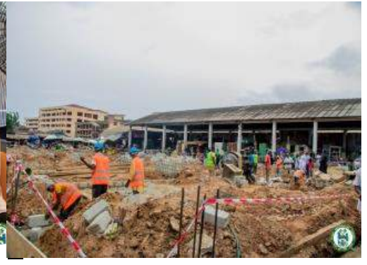
Modernization of Makola Market sheds progressing steadily
