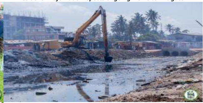
Ongoing desilting of drains in Accra
