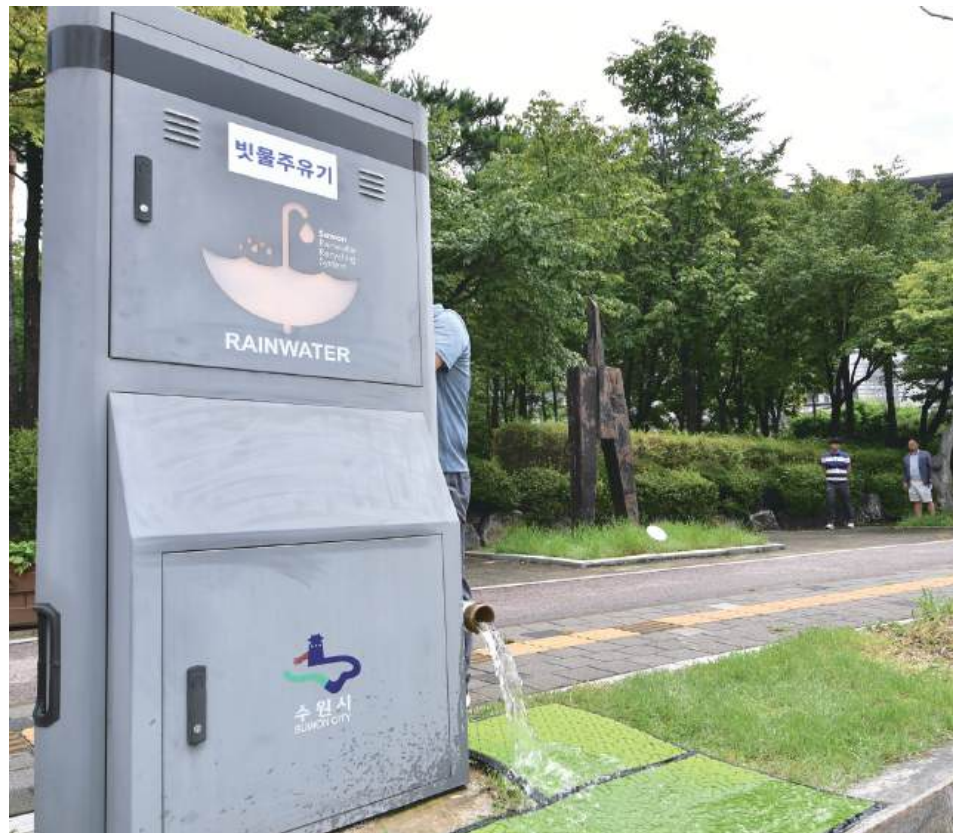
Rainwater station installed near the World Cup Stadium
