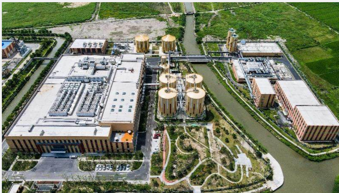
Figure 17 Wet Waste Incineration Plant of Tianma Zero-waste Low-carbon Environmental Protection Industrial Park
