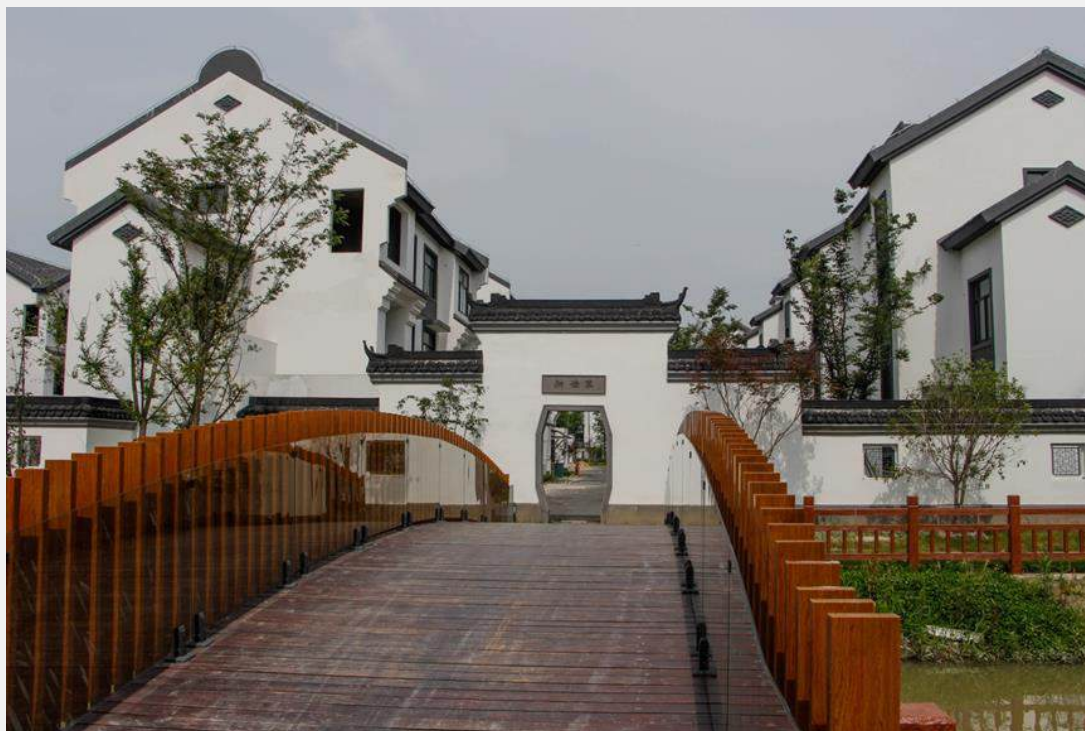
Figure 15 Village Appearance after Rectification
