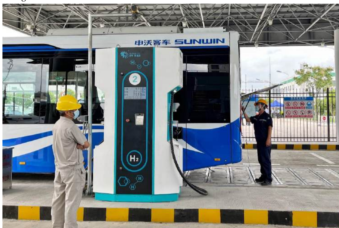
Figure 8 Fengxian hydrogen refueling station for hydrogen fuel cell buses
