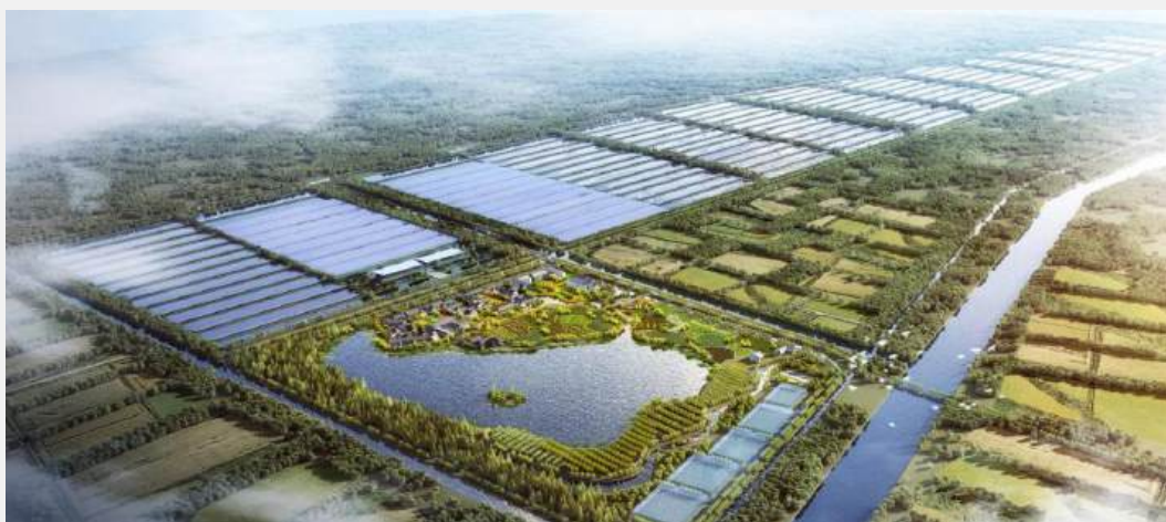
Figure 9 A picture of Fishery-Photovoltaic Complementary Project in Chongming District
