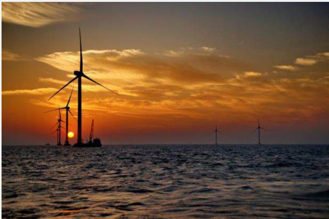
Figure 10 Offshore Wind Farm near Donghai Bridge, Shanghai
