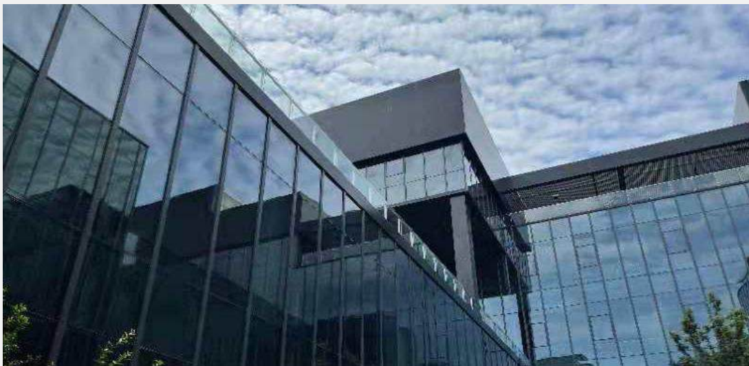
Figure 9 Shanghai's First Thin-film BIPV Building Triumph Robot Intelligent Equipment R&D Center
