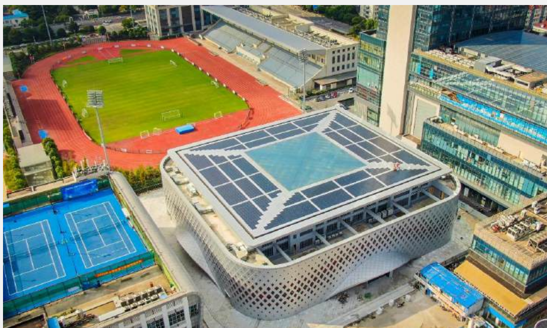
Figure 7 Rooftop Photovoltaic Power Generation Project of Songjiang Stadium
